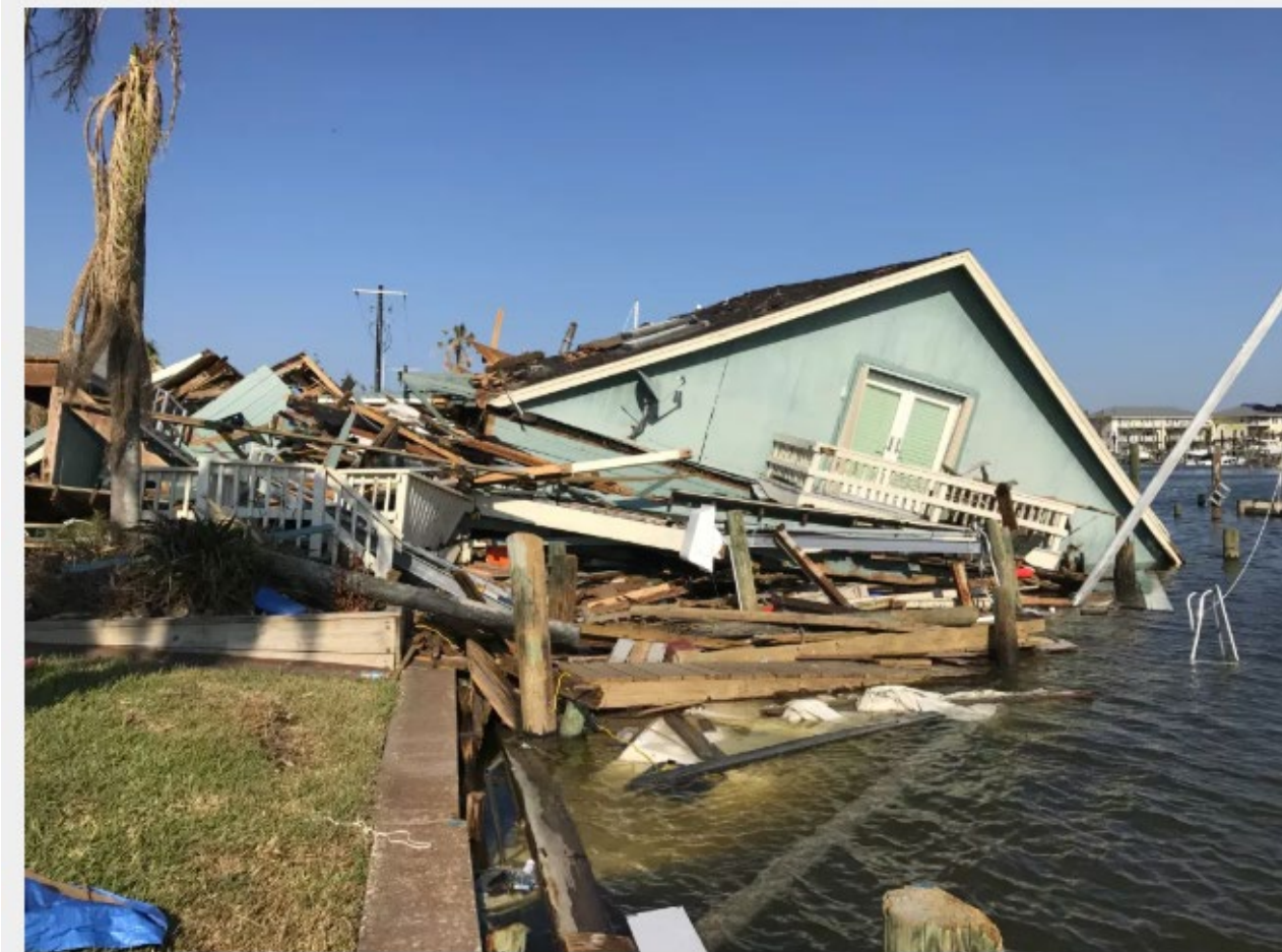
A TWO-STORY CONDOMINIUM COLLAPSED IN HIGH WINDS WHEN STORM SURGE UNDERMINED ITS FOUNDATIONS.
