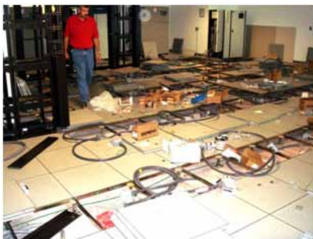
Courthouse IT server facility on six-inch raised floor during installation.
