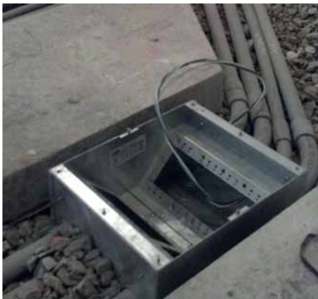
A floorbox and conduit runs placed in a trenched concrete floor.
