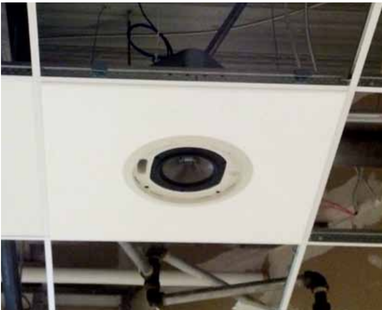
A ceiling-mounted loudspeaker installed during construction.
