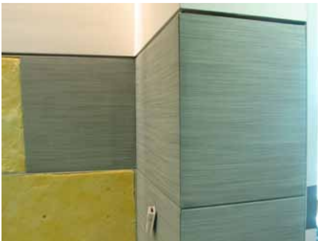
Acoustical wall panel installation, Manatee County Courthouse.
