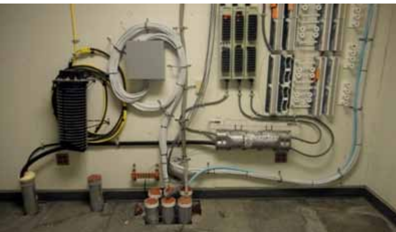
A typical demarcation room. The optical fiber and cables coming out of the floor conduits are connected outside of the building.
