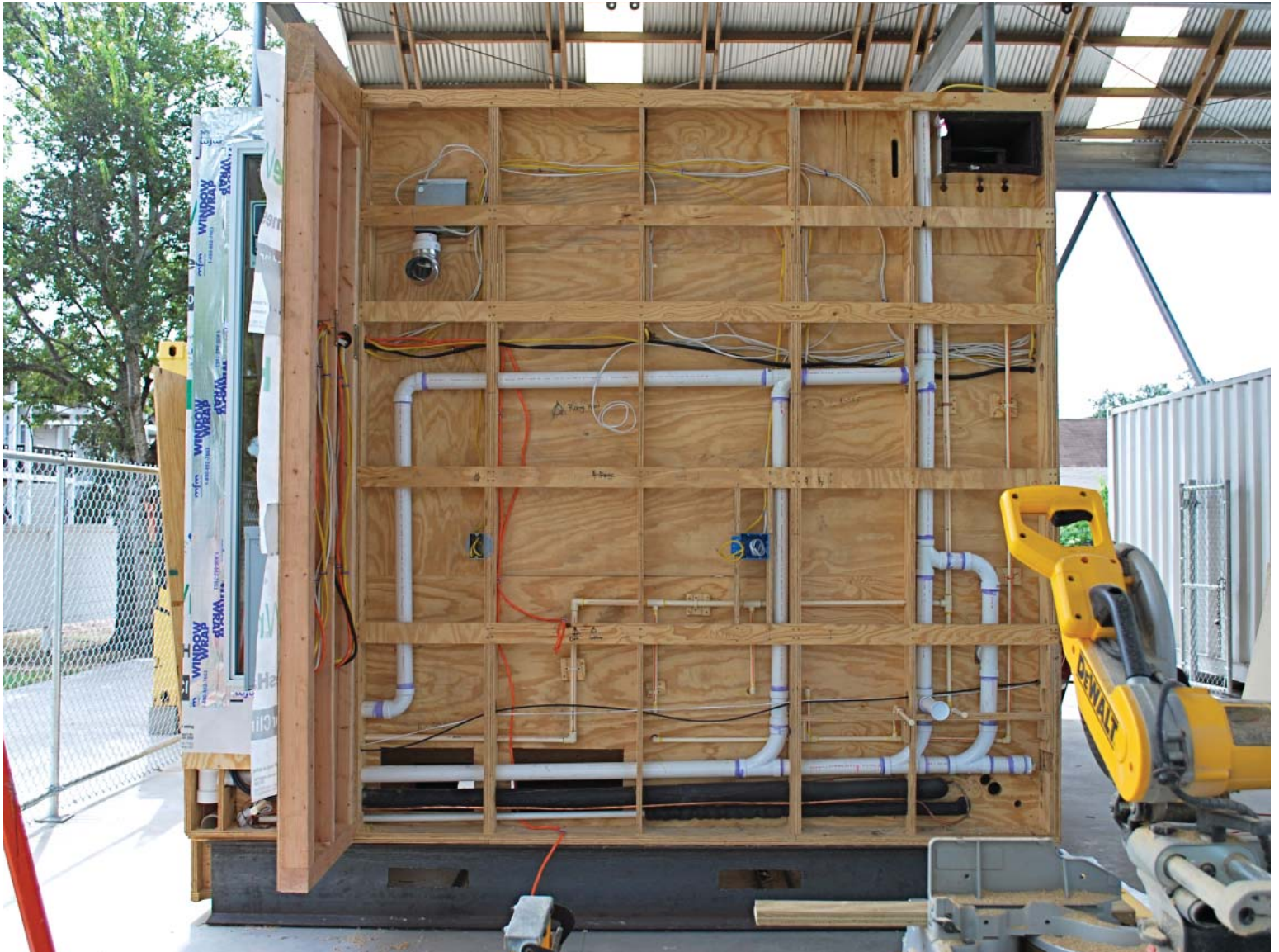
ROUGH IN : TRADESMEN BEGIN TO ROUGH IN THE SYSTEMS THAT OPERATE IN THE INHOUSE OUTHOUSE
