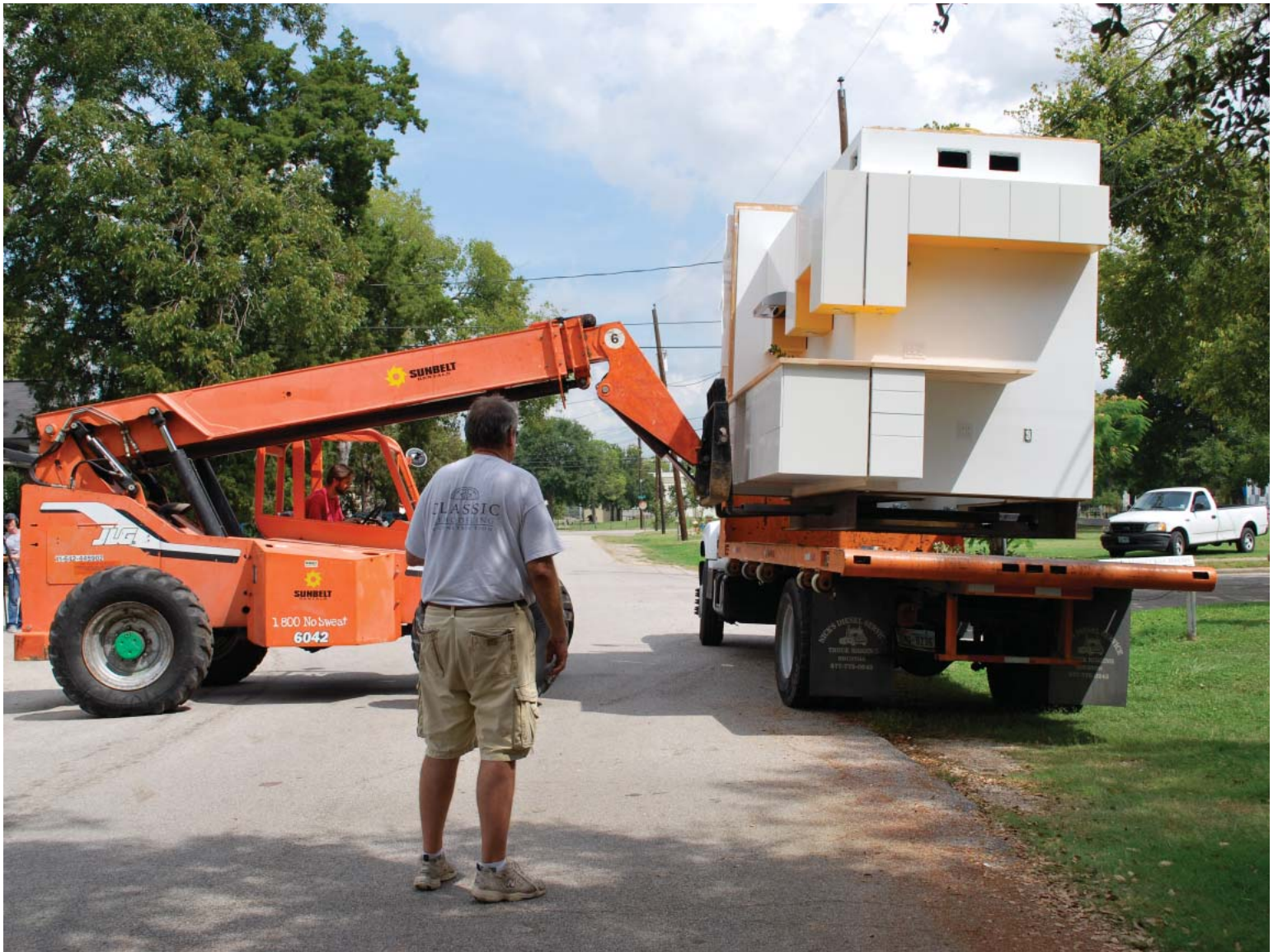
THE MOVE : ONCE AT SITE, THE FORKLIFT IS READY TO ACCOMPLISH THE MAJOR POSITIONING
