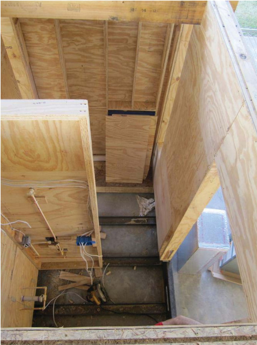
BATHROOM : INTERIOR VIEW OF BATHROOM ROUGH IN, IN PROGRESS
