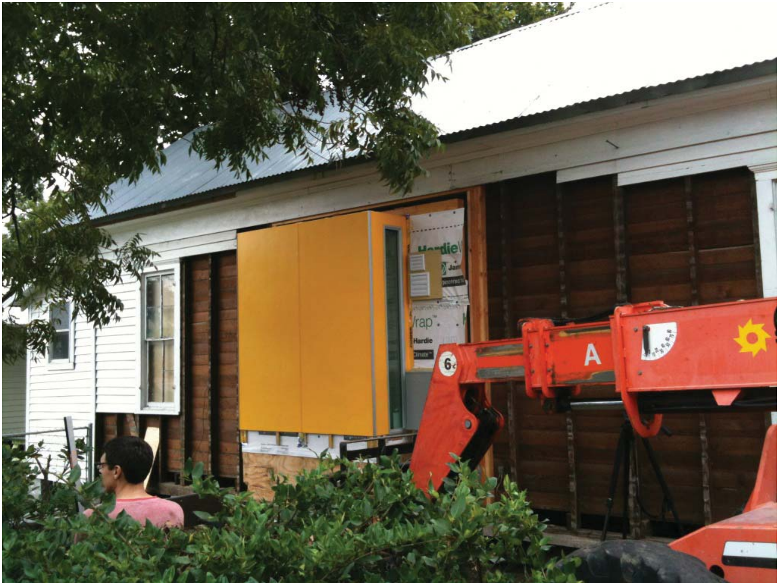
THE MOVE : ONCE IN PLACE, COME-ALONGS ARE USED TO CRANK THE PROTOTYPE INTO THE HOUSE
