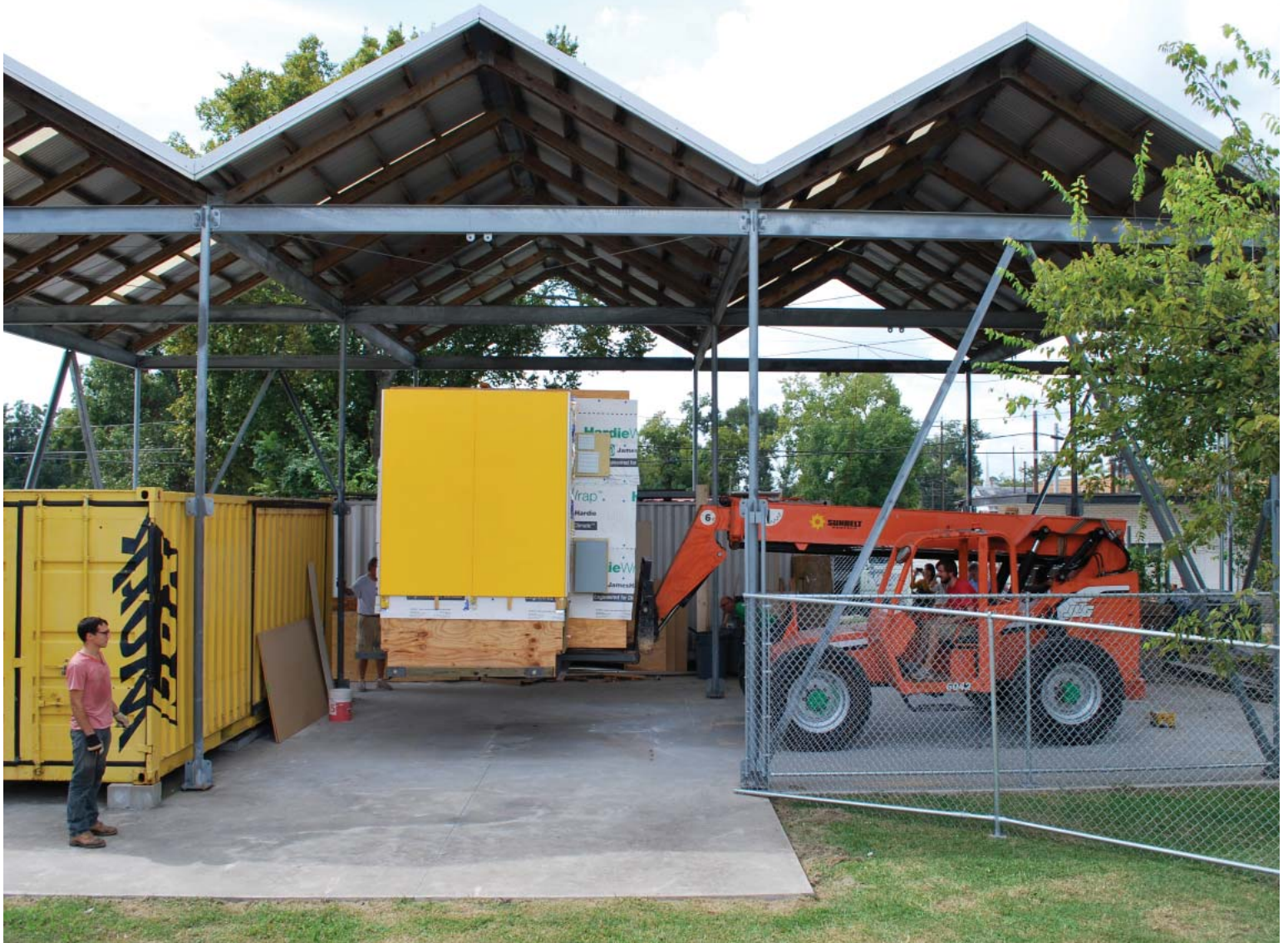
THE MOVE : THE PROTOTYPE IS LIFTED SO THAT THE FLATBED CAN BE MOVED UNDER IT
