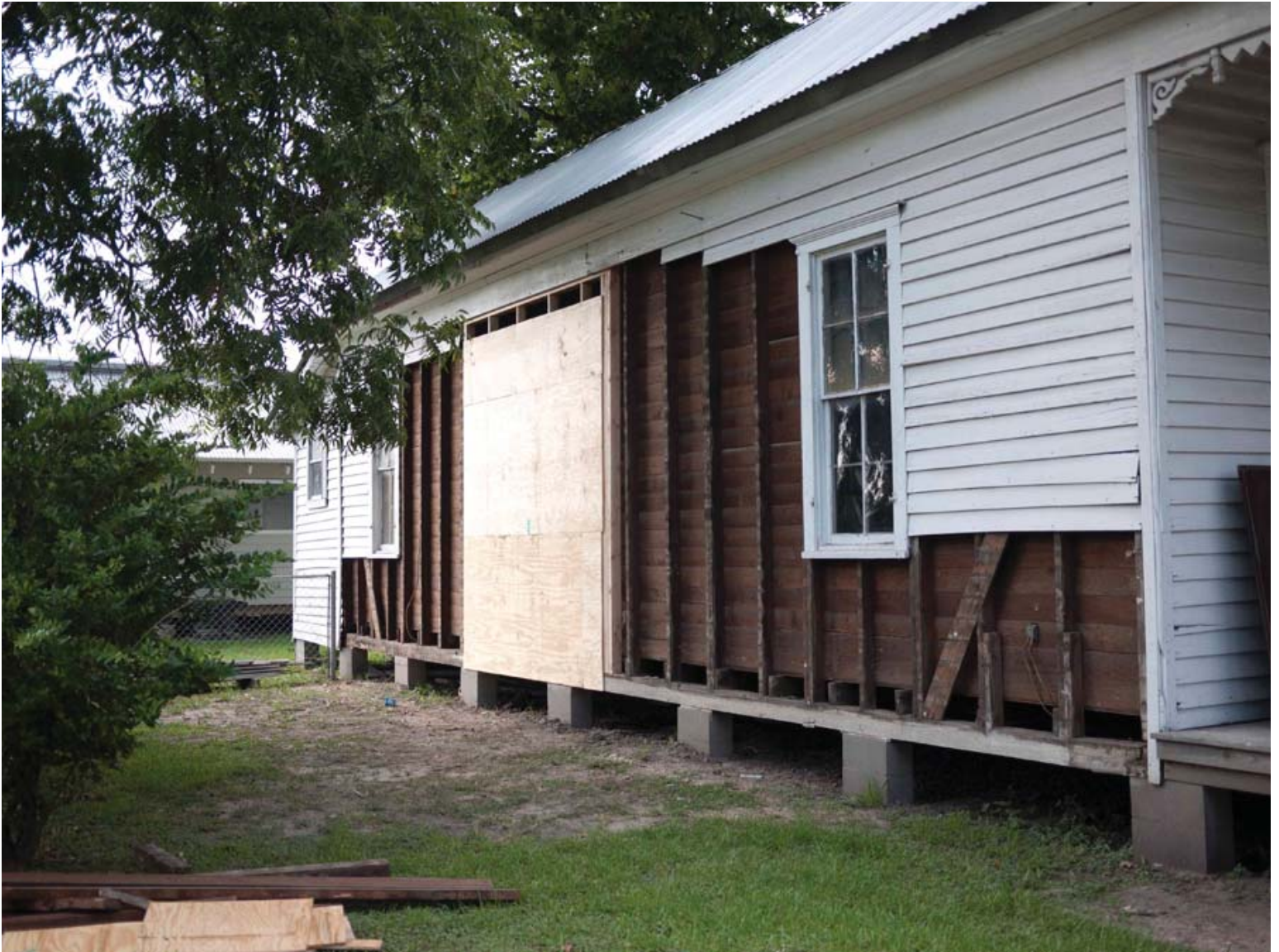
SITE PREPARTION : A NEW STRUCTURAL HEADER IS ADDED AS WELL AS A TEMPORARY SHORING WALL
