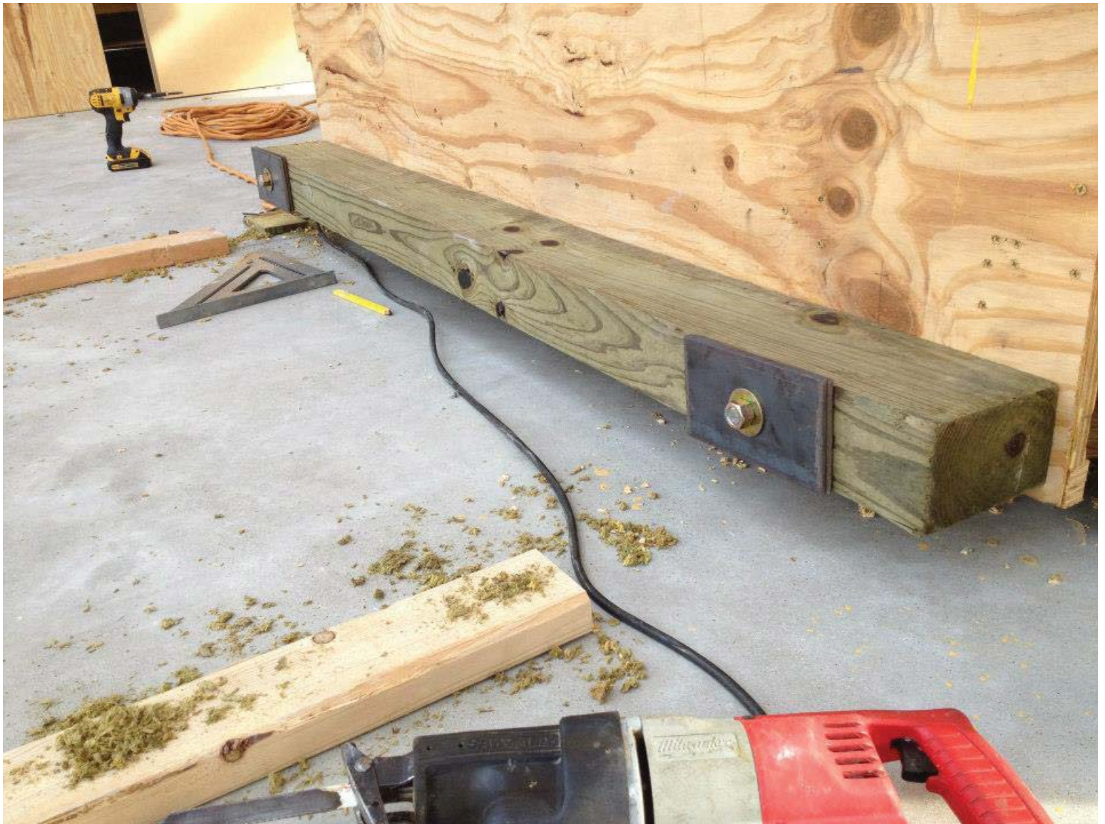
PREPERATION : A 4X6 MEMBER IS USED AS A BRACE
