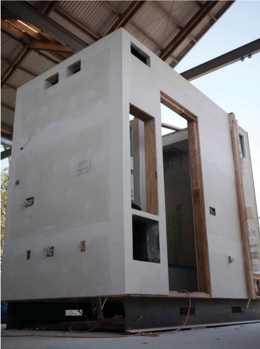
DRYWALL : MANY COATS OF JOINT COMPOUND ARE NECESSARY
