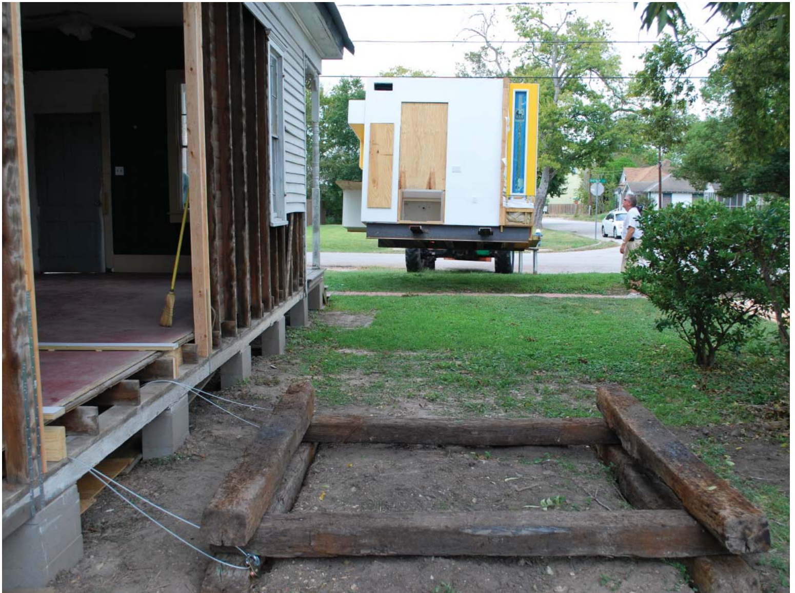
TRAY SYSTEM : A CRUDE SYSTEM OF RAILROAD TIES SERVES AS A BASE FOR THE DELIVERY TRAY
