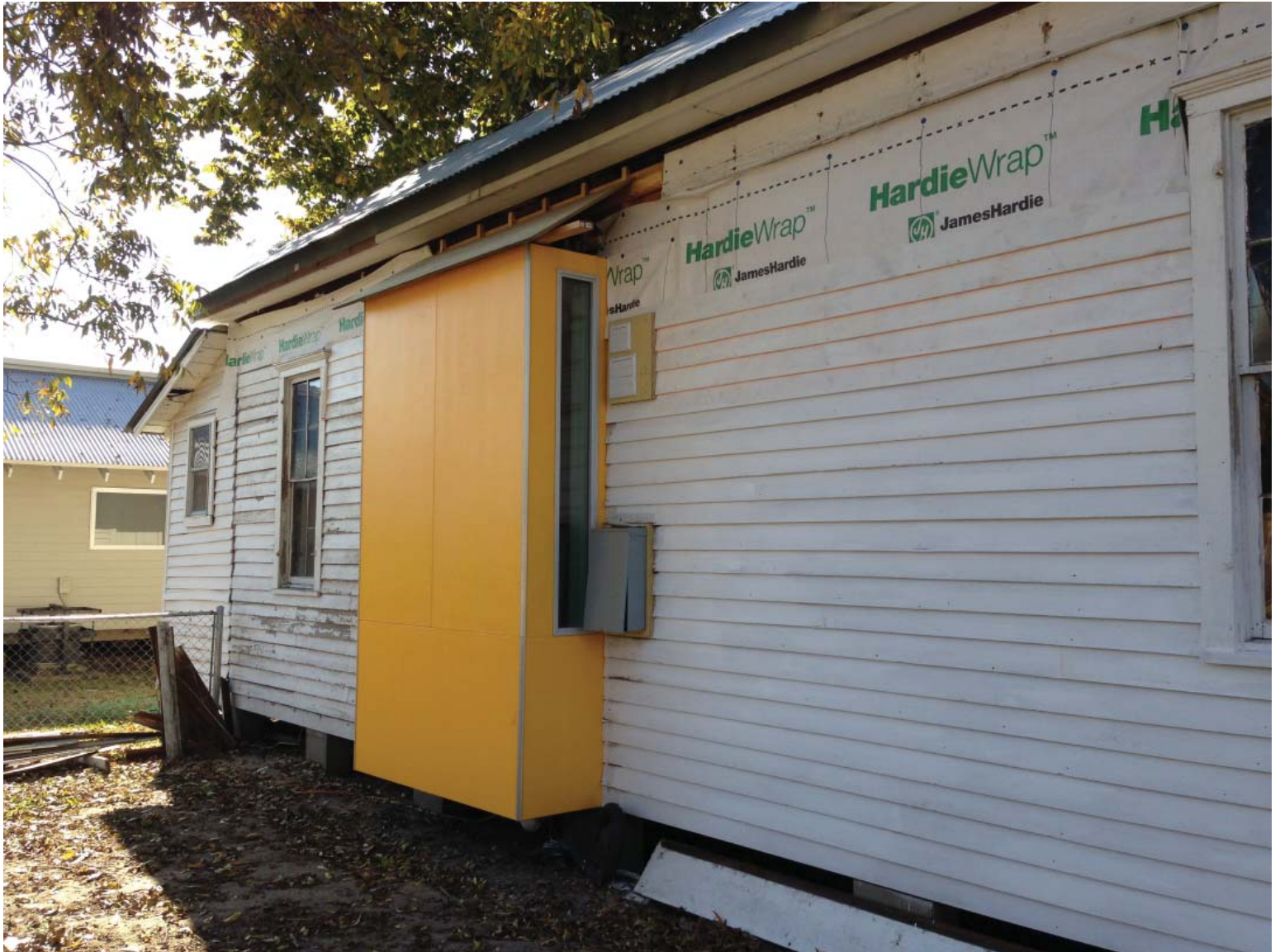
IN SITU : INHOUSE OUTHOUSE PROTOTYPE INSTALLED WITH NEW INSULATION AND REUSED SIDING
