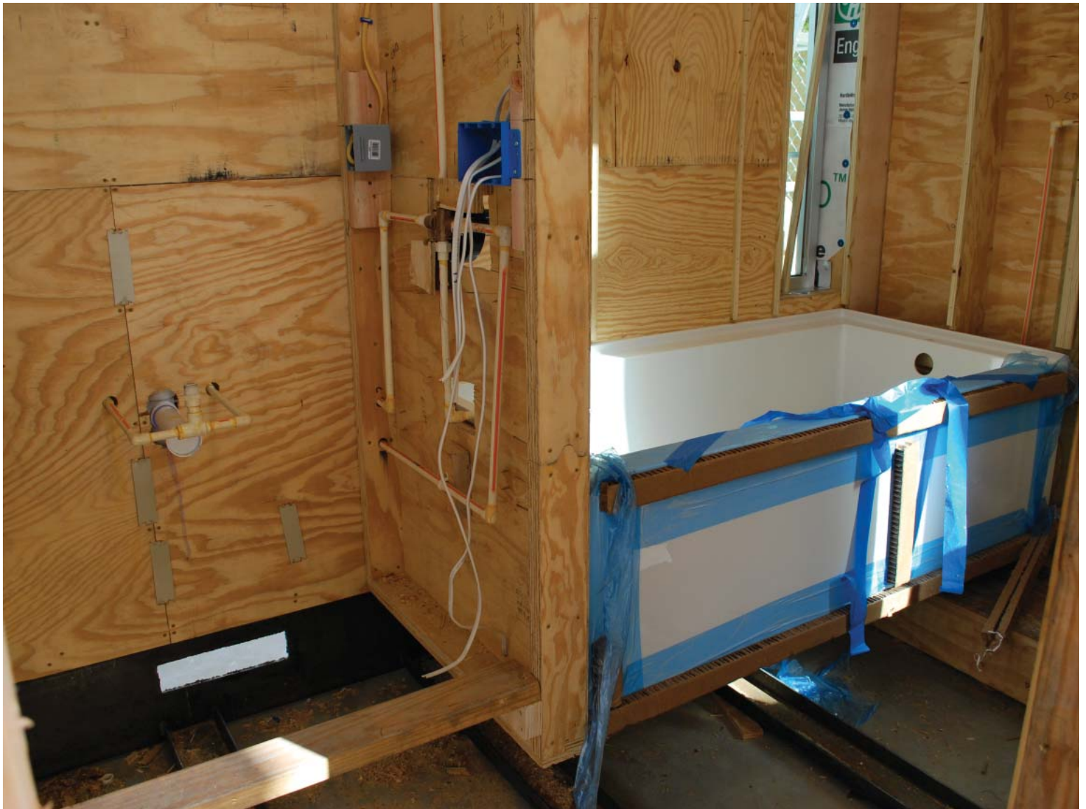
BATHROOM : VANITY (LEFT) ROUGH IN; TUB SET (RIGHT)
