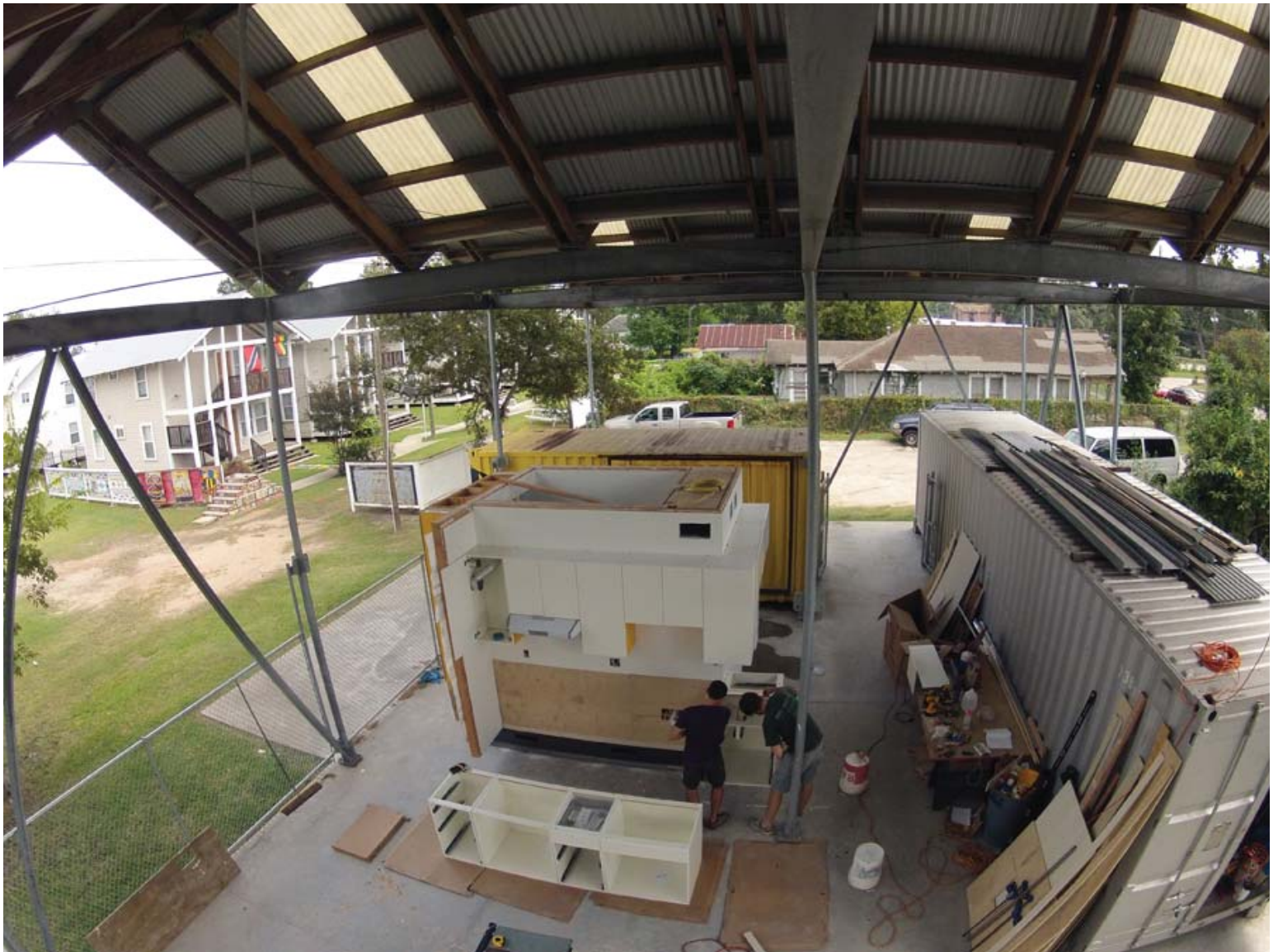
CABINETS : BASE CABINETS ARE ADDED AND HUNG FROM THE STRUCTURAL FRAME AS WELL
