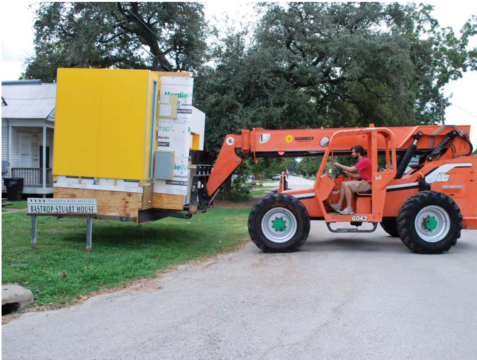
THE MOVE : THE INHOUSE OUTHOUSE SPECIFIES AN ALL-TERRAIN FOKRLIFT FOR ROUGH SURFACES
