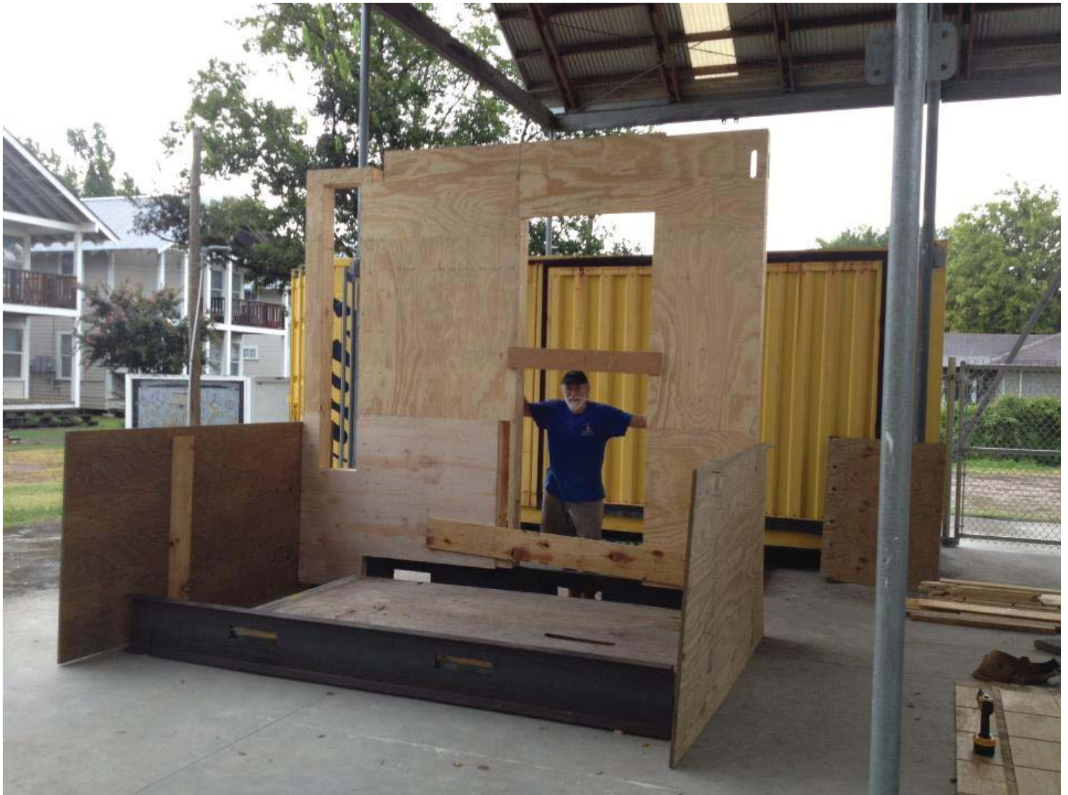
WALL ASSEMBLIES : AS A KIT OF PARTS, THE WALLS FOR INHOUSE OUTHOUSE ASSEMBLY QUICKLY
