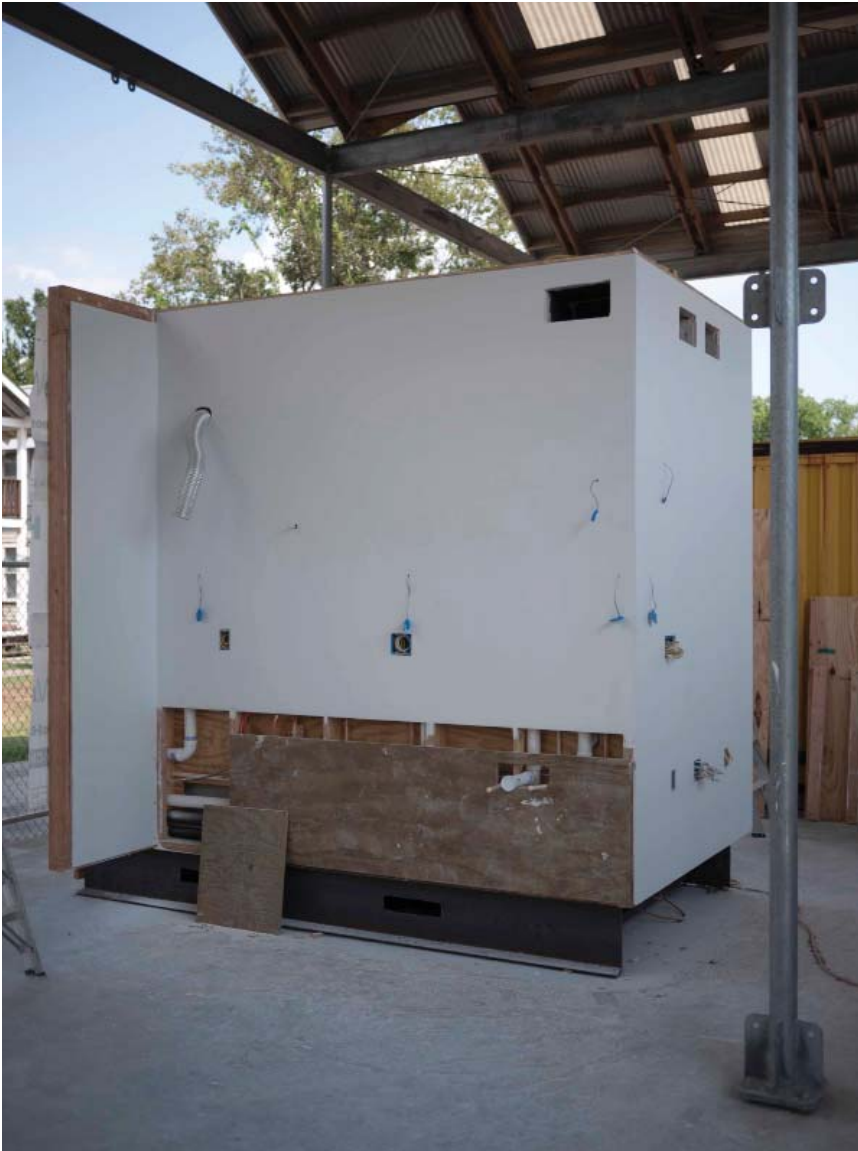
PAINT : THE LAYERS OF JOINT COMPOUND ALLOW FOR A SMOOTH FINISHED SURFACE FOR PAINT
