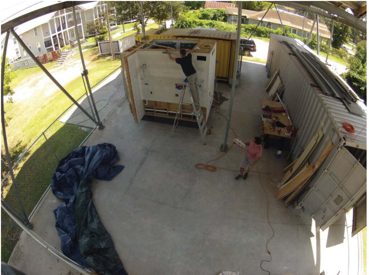
DRYWALL : ONCE COMPLETELY HUNG, JOINT TAPE AND JOINT COMPOUND ARE APPLIED TO SEAMS
