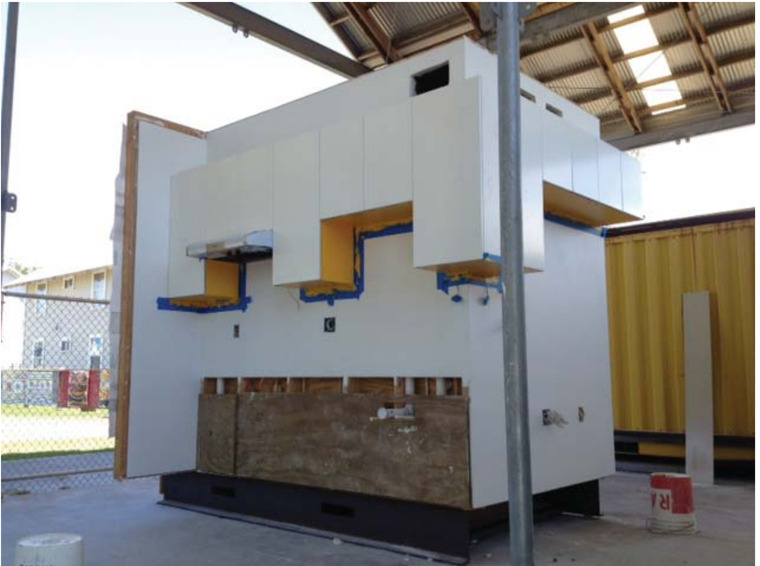
CABINETS : FOLLOWING MULTIPLE COATS OF PRIMER AND PAINT, WALL CABINETS ARE HUNG
