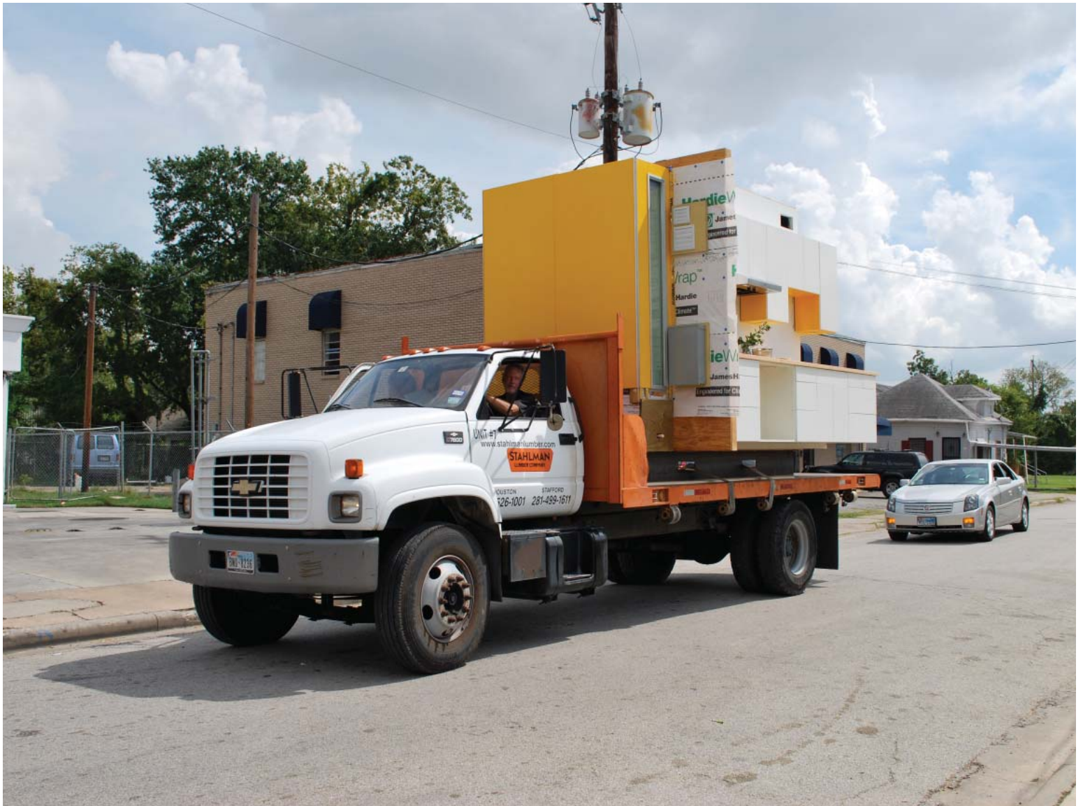
THE MOVE : THE PROTOTYPE, AT 8'-6" WIDE IS MEANT TO SIT ON A TRUCK WITHOUT WIDE LOAD STATUS
