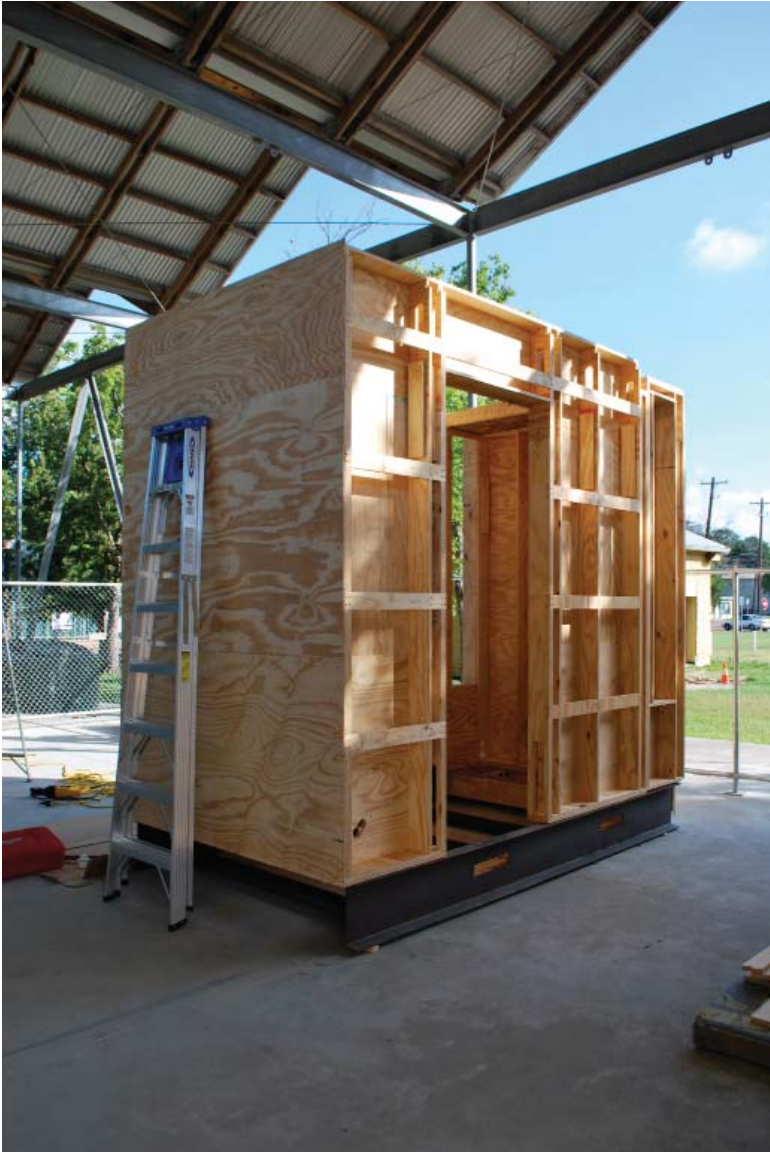
STRUCTURAL SHELL : COMPLETED INHOUSE OUTHOUSE STRESSED STRUCTURAL PLYWOOD SHELL
