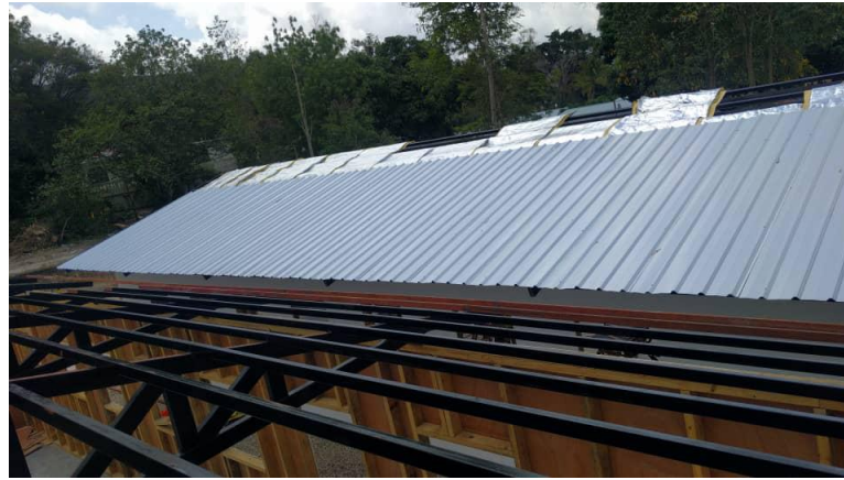
14: Install Roofing
