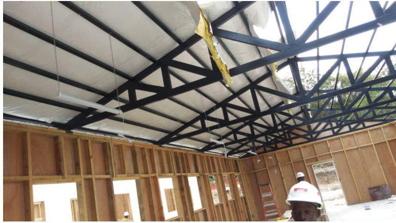
13: Insulate Roof
