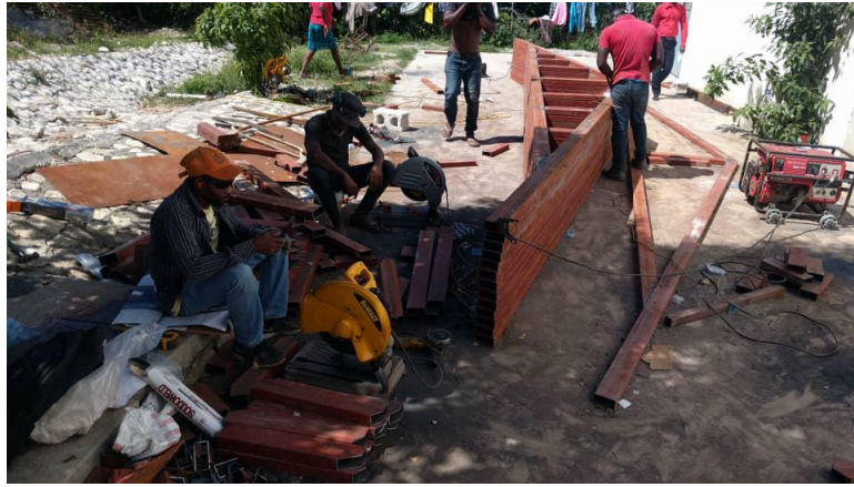
7: Assemble Trusses
