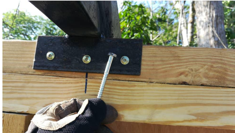
11: Bolt Truss Plates
