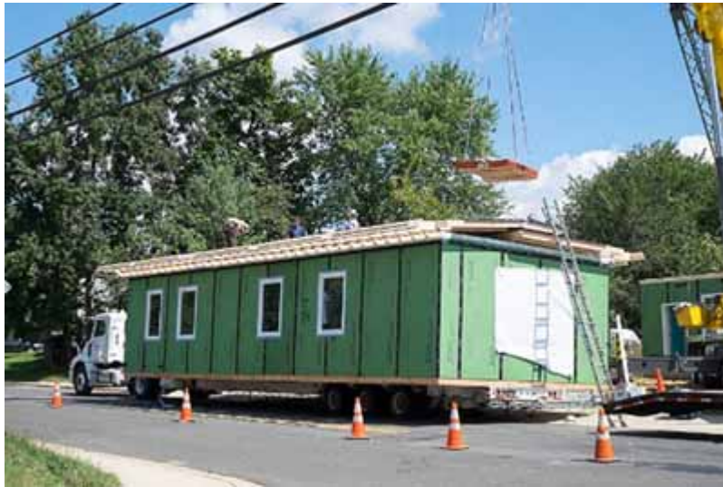
Second story unit as it arrived on site with the roof folded and without the eave overhangs. Photo credit: David Peabody.
