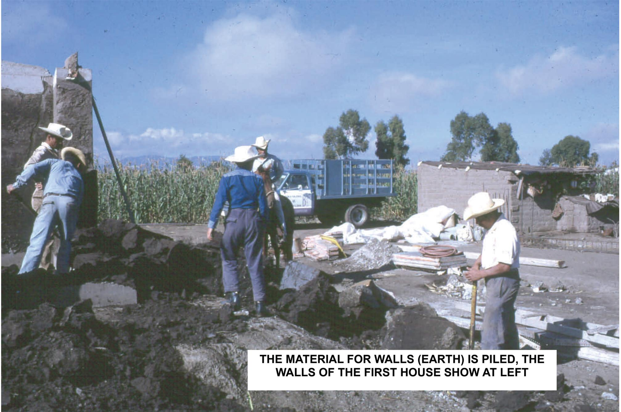
**THE MATERIAL FOR WALLS (EARTH) IS PILED, THE WALLS OF THE FIRST HOUSE SHOW AT LEFT**
