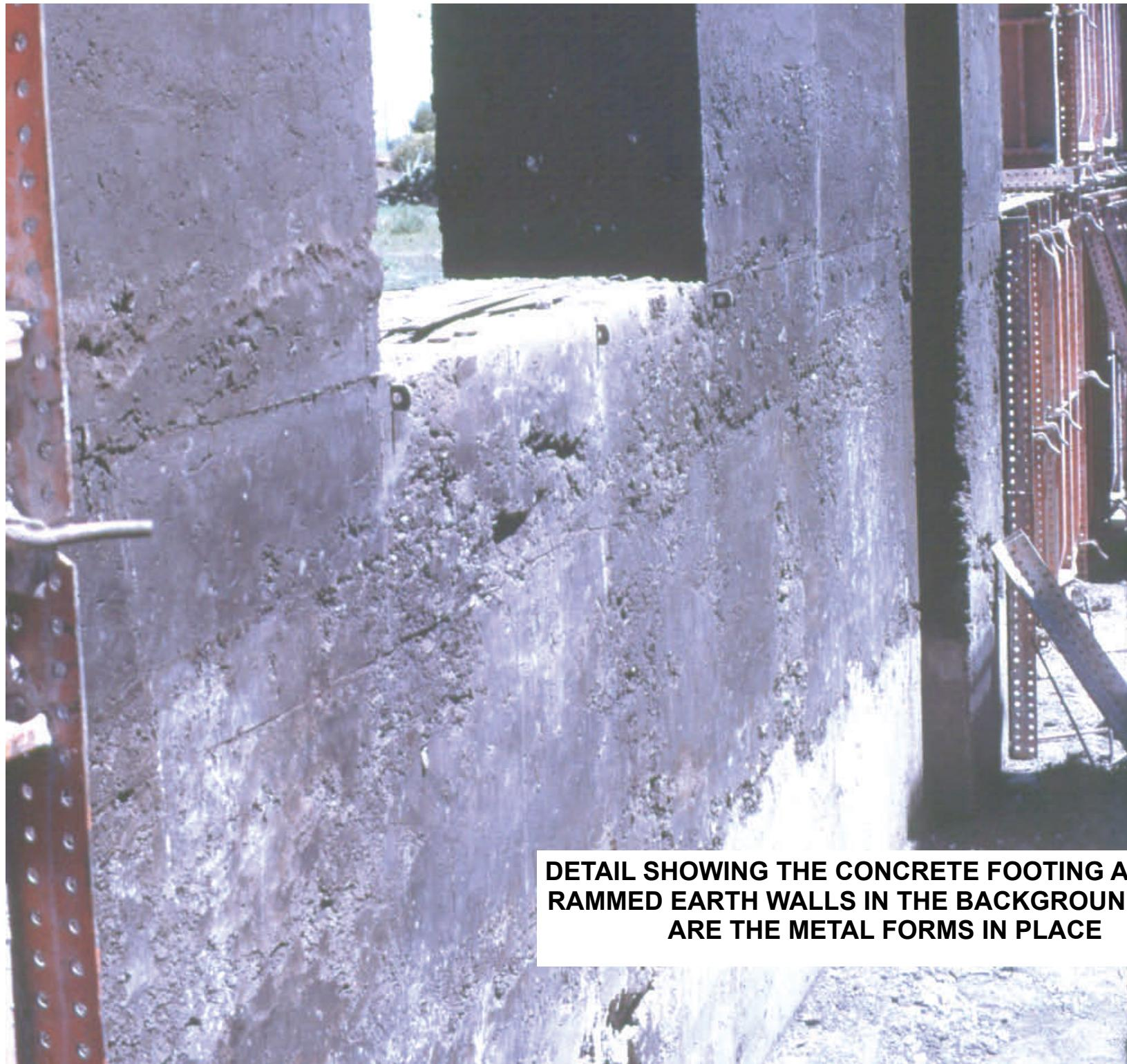
**DETAIL SHOWING THE CONCRETE FOOTING AND THE RAMMED EARTH WALLS IN THE BACKGROUND STILL ARE THE METAL FORMS IN PLACE**
