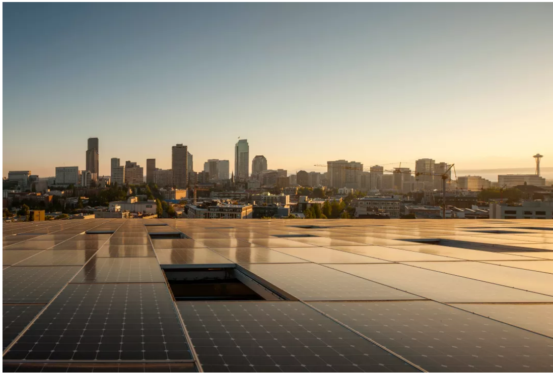
The roof of the Bullitt Center in Seattle, the 2016 COTE Top Ten recipient. Designed by Miller Hull, it features 575 pv panels on the roof at 425 watts per panel. | PHOTO: Nic Lehoux
