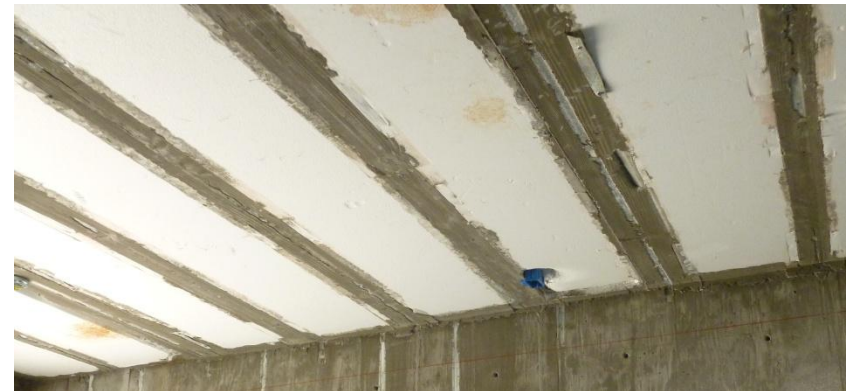
View of roof steel reinforcement and EPS insulation
