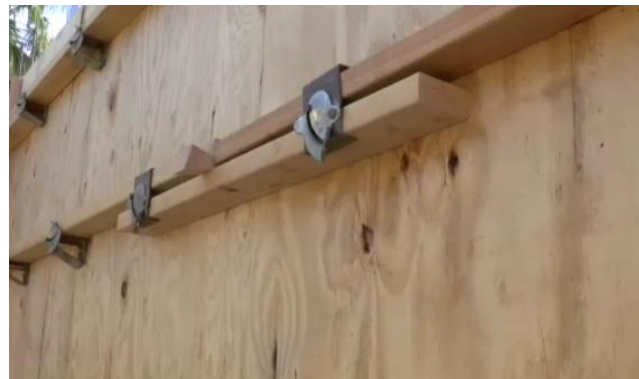
Jahn "C" brackets are used in scabbed joints for long formwork for walls.
