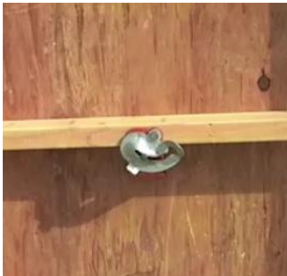
2x4 wale hold by a Jahn "A" bracket hold by a Brigade Snap tie short end, hex-head.
