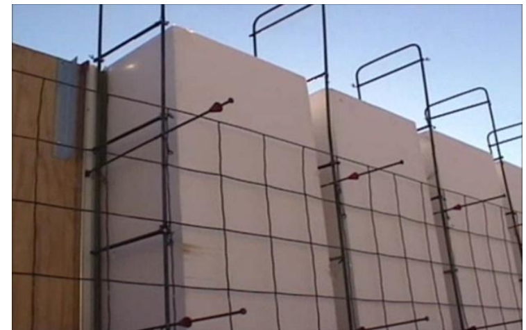
Actual photo of formwork with nailer and angles, EPS blocks Snapties, and diaphragm wire mesh.
