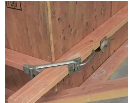
Jahn Corner lock used at outside corners to secure 2x4 wales
