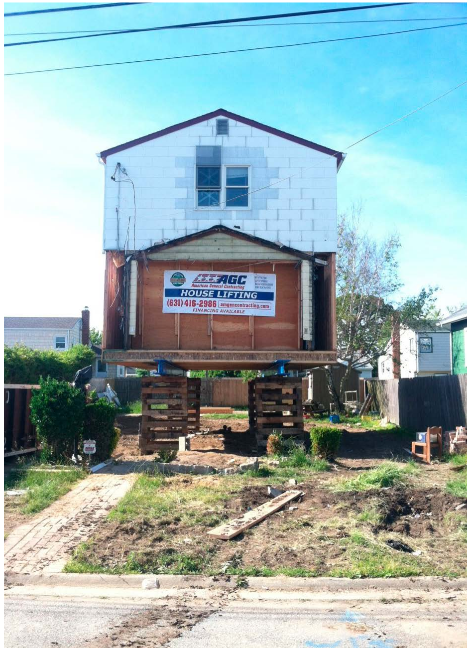
Above: A house lift on Long Island. Image courtesy Daniel Horn. Above left: 5 building blocks of resilient reconstruction. Image courtesy of ORLI.
