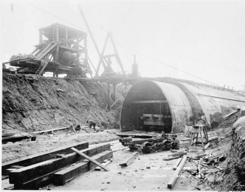
Typical Cut and Cover Section
