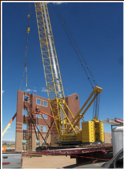
Precast/brick composite panels erection
