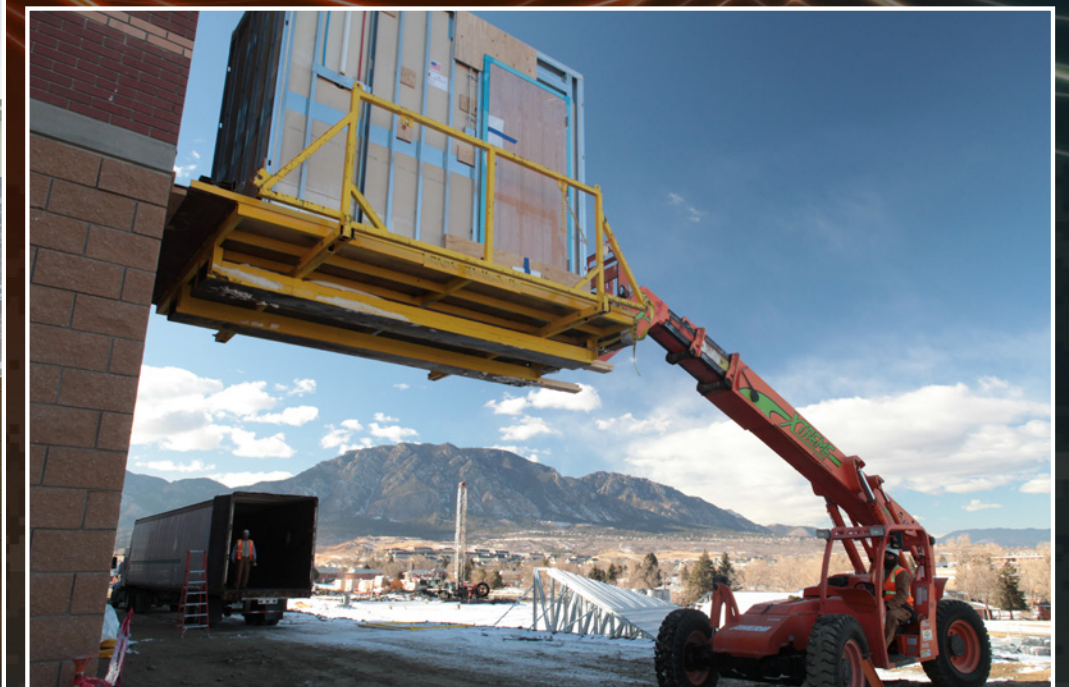
Top left: Model based rendering of courtyard. Top Right: Front Entry 'knuckle' model based design rendering. Middle: Prefabricated Roof Truss on the ground. Middle Right: Prefabricated Roof Truss lifted into place. Bottom Left: Common space- model based rendering. Bottom Right: Bathroom module installation process.
