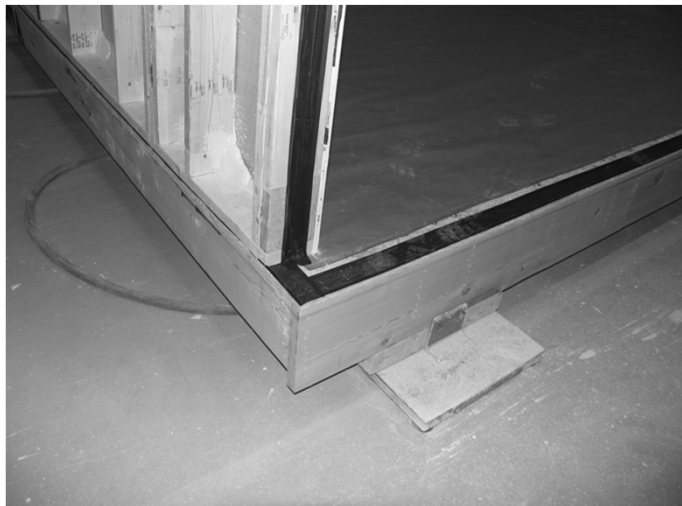
EPDM gasket at floor and wall intersections
