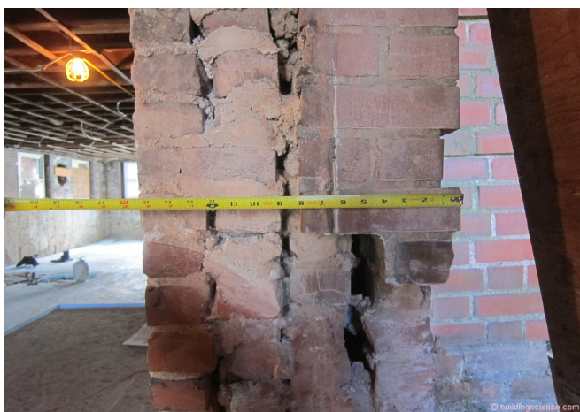
Photograph 3 – Brick Wall Section: Solid mass walls are not typically solid. Let me repeat...solid mass walls are not typically solid.
