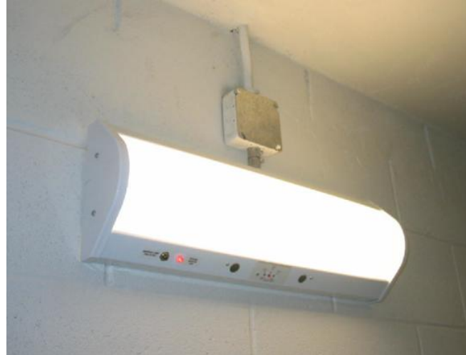
Motion Sensor Stairwell Light
