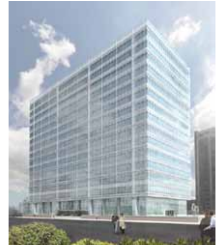
4. OVER-CLAD Existing Facade
