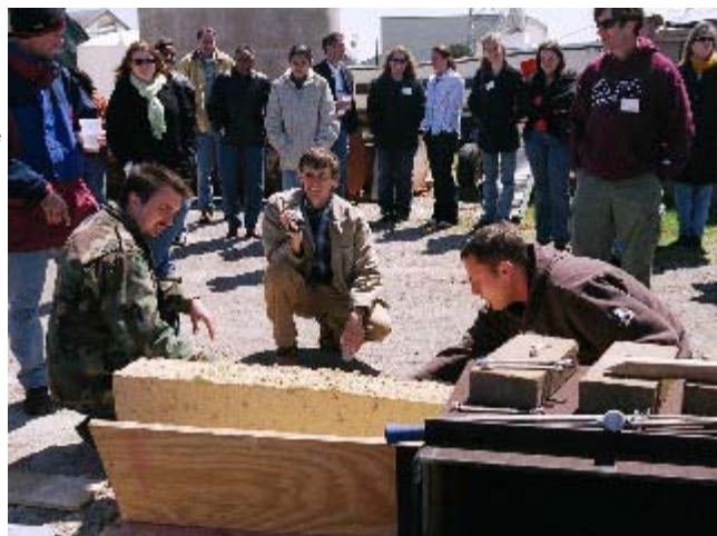
Students demonstrate rammed earth construction at Texas A&M symposium. Photo by Professor Richard Burt.
