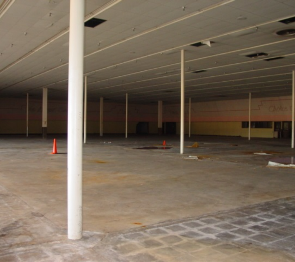
EXISTING BIG BOX STRUCTURE CLEARANCE OF 21'-0" A.F.F.
