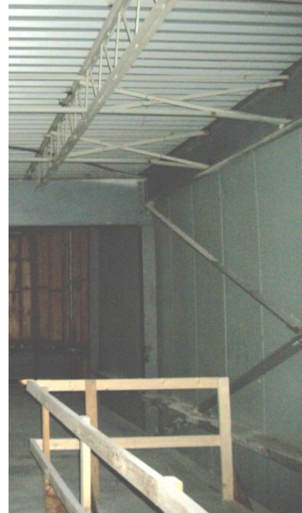
EXISTING STRIP MALL STRUCTURE CLEARANCE OF 12'-6" A.F.F.
