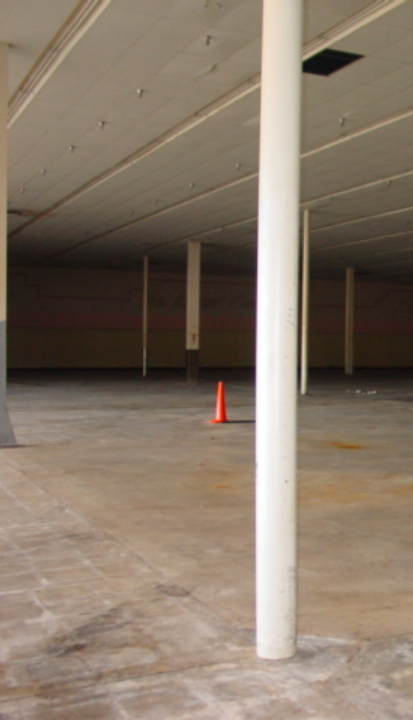
EXISTING BIG BOX STRUCTURE CLEARANCE OF 21'-0" A.F.F.
