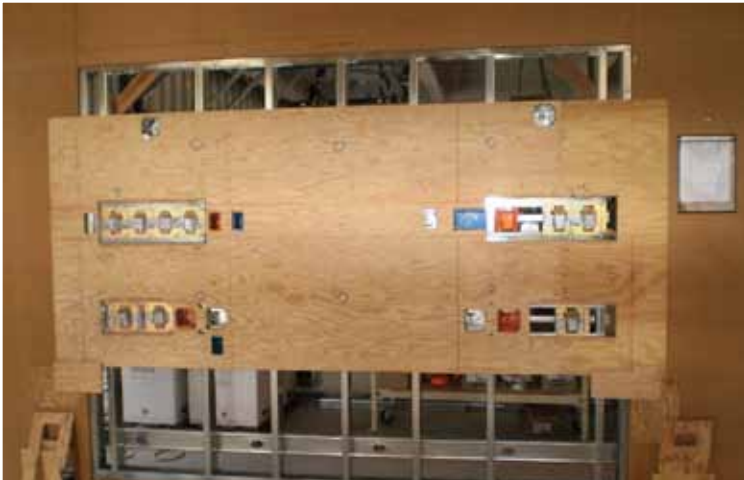
CNC prefabricated head wall template.
