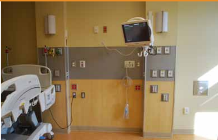
Actual Photo: Completed CNC prefabricated headwall installed in patient room.
