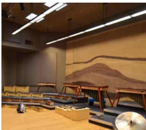
Image 23: The rammed earth wall provides thermal protection for the music and dance rooms.
