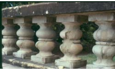
Figure 3: Deteriorated balusters at Stanford's Main Quad Balustrades, 2004 (Stanford University)
