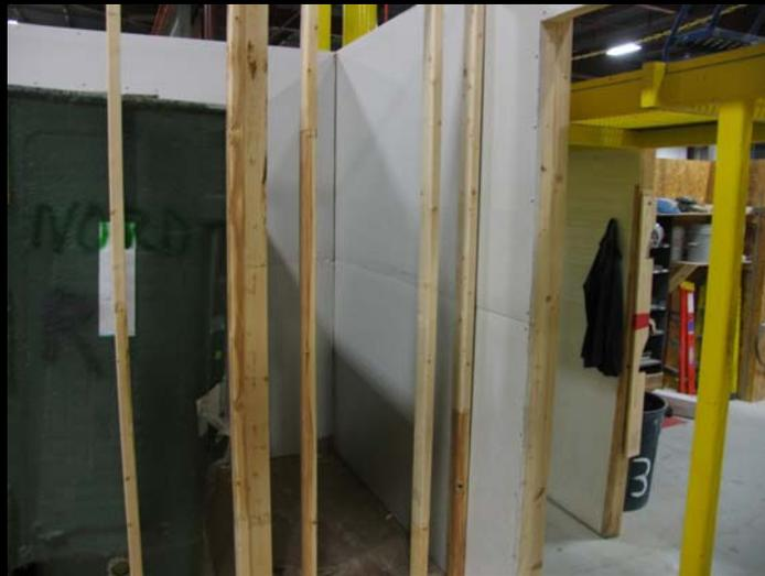
Foam sprayed on sheetrock joints
