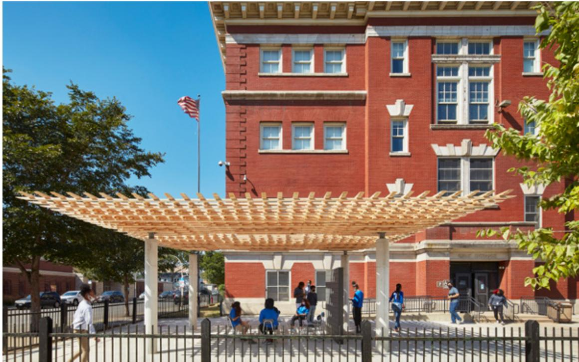
timber reduces material use by nearly 50% compared to cross-laminated timber panels. As a project, the pavilion effectively demonstrates ways to minimize timber consumption and overall carbon footprint when used to construct an entire building.
