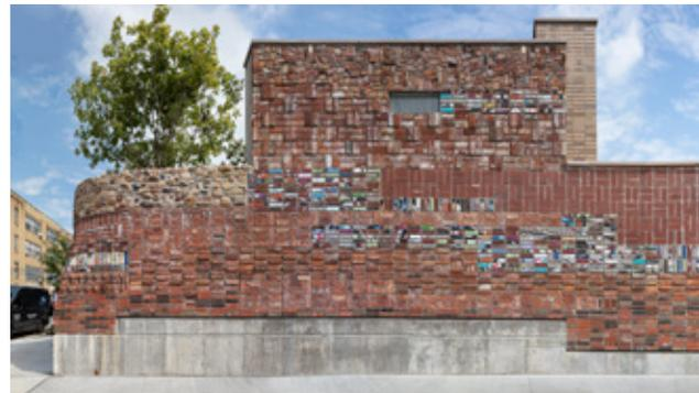
materials, stones tumbled and smoothed by a retreating glacier, being brought to the site during the last ice age. Masonry from the site's warehouses and cold storage facilities was gathered, scraped by hand on-site, and carefully cataloged. A poured concrete wall served as a blank canvas for an original composition that showcases the site's material history in an impressionistic manner.
