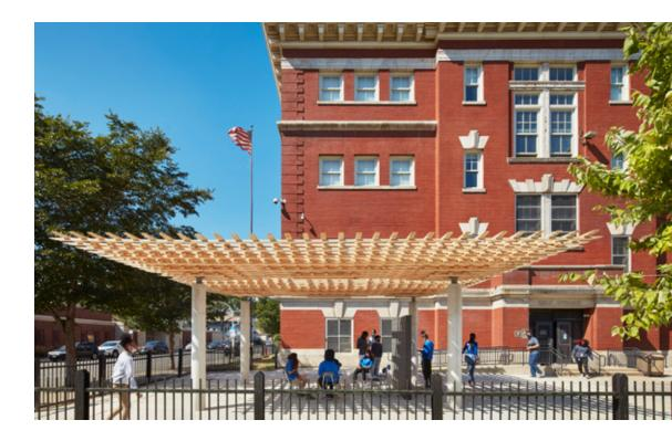
timber reduces material use by nearly 50% compared to cross-laminated timber panels. As a project, the pavilion effectively demonstrates ways to minimize timber consumption and overall carbon footprint when used to construct an entire building.
