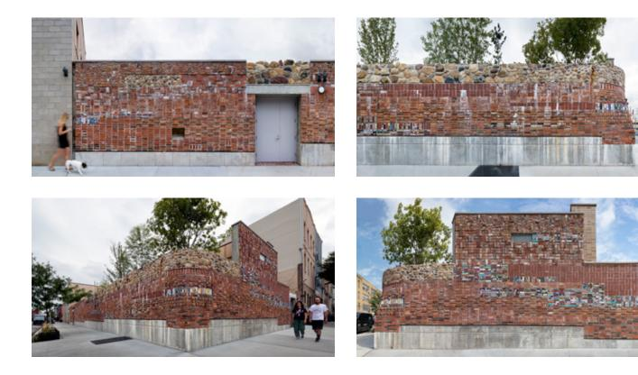
materials, stones tumbled and smoothed by a retreating glacier, being brought to the site during the last ice age. Masonry from the site's warehouses and cold storage facilities was gathered, scraped by hand on-site, and carefully cataloged. A poured concrete wall served as a blank canvas for an original composition that showcases the site's material history in an impressionistic manner.
