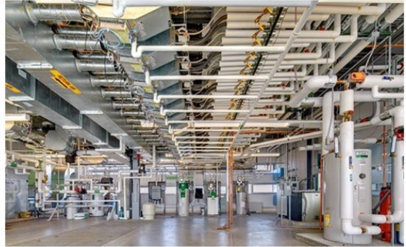
Researchers controlled indoor environmental quality from a space underneath the testing environment to simulate conventional and green building conditions.
