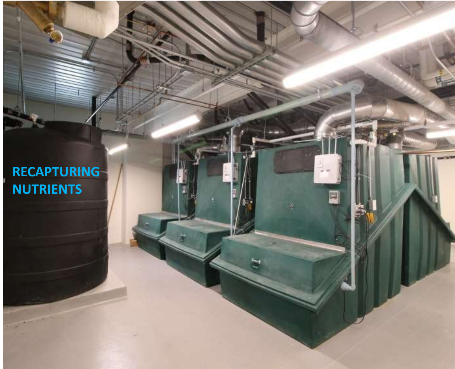
Composting Toilets with Foam-Flush fixtures and leachate collection
