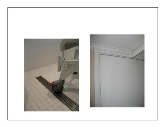
Think about the functional details. We chose to position the drain at the front edge of the shower area to create a single slope pitch from the back wall of the shower by adding to the height of the subfloor and not cutting or reframing to create a recess.
