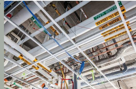
Installed systems using pre-installed anchors. Subcontractors had confidence that the cast-in anchors would be where they needed them to be weeks or months later.
