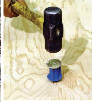
Installation of the MEP system anchors from the top of the form was a tremendous cost benefit for the owner.
