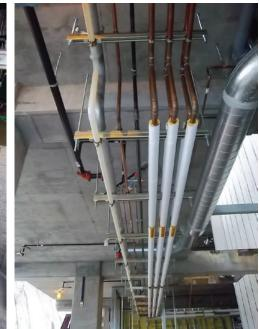
Installed duct work and pipe racks with connection to other pipe rack sections.
