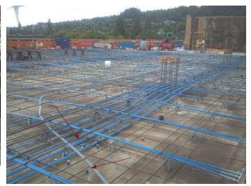
Anchors installed from the top of the forms. These were installed with information from the model and input into a survey program.
