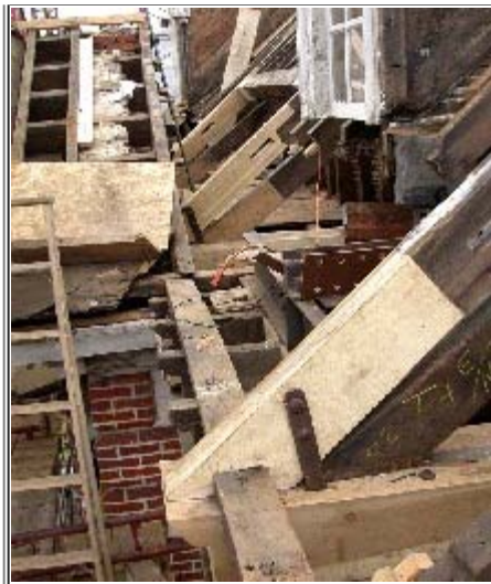
Photo: Courtesy Philadelphia Museum of Art View of heavy timber truss repair splices using in-kind wood species members attached with concealed steel plates in structural epoxy matrix.
