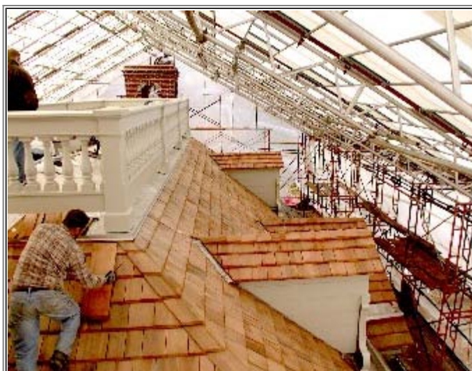
Photo: Courtesy of Philadelphia Museum of Art Mount Pleasant roof restoration nearing completion under complete scaffolding cover.
