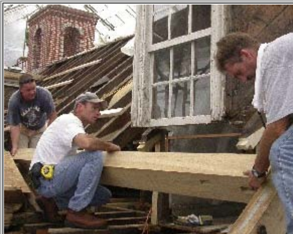
Photo: Courtesy of Philadelphia Museum of Art Carpenters install a new 7" x 7" poplar purlin beneath the northeast dormer of Mount Pleasant Mansion.
