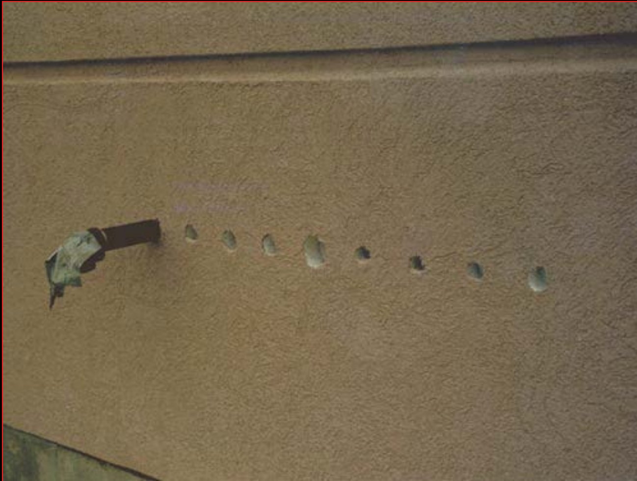
Result of 'zero' coordination for penetrations
