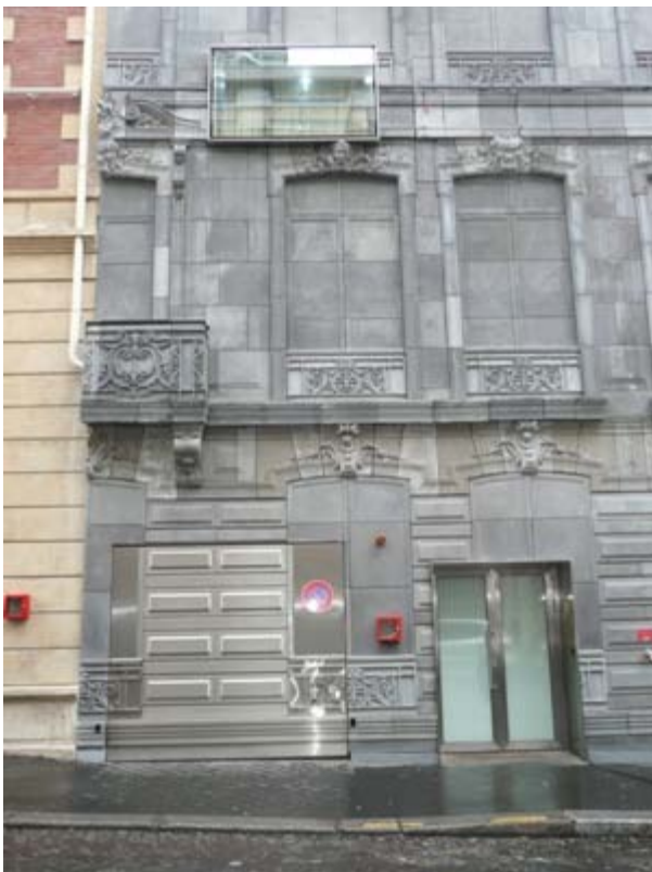
Hôtel Le Fouquet Paris. Detail of molded concrete panels. Photo: Wendy Hillis, AIA. February 2008.
