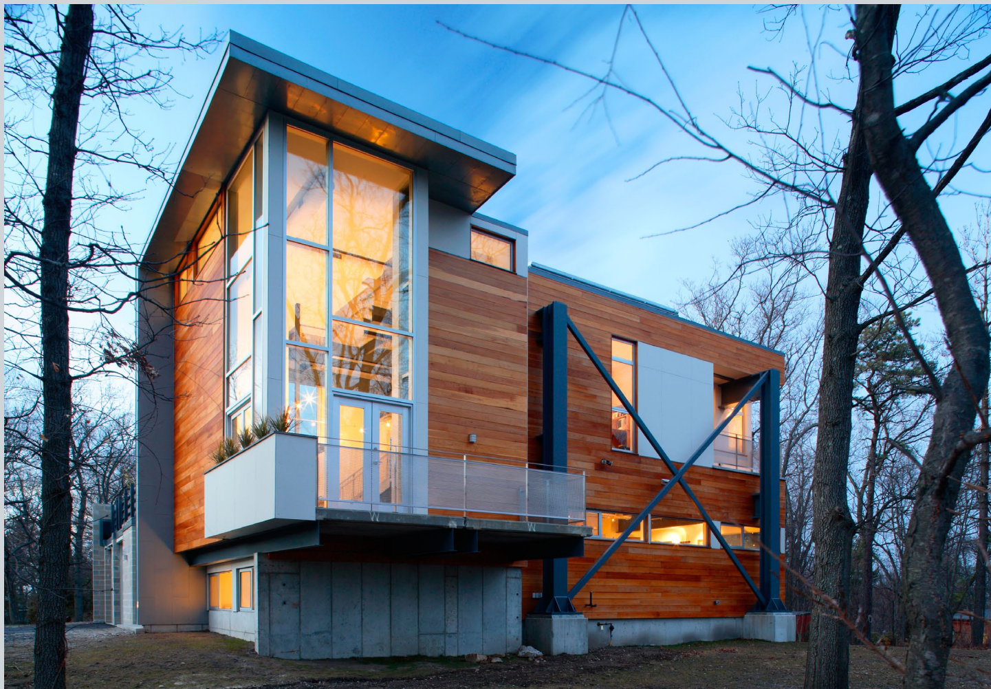
Above: Big Dig House utilizes salvaged infrastructure for its structural system. Right: Songpa Micro-Housing incorporates a multifunctional screen. Images © SsD.
