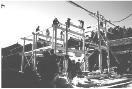
Fig.1-8 New Naxi courtyard under construction
