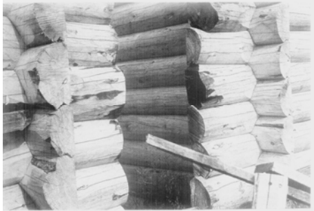
Fig.4-3 Stacked log construction
