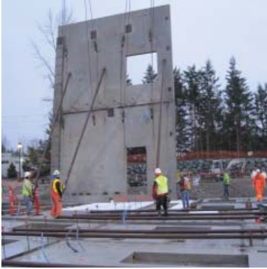
TILT-UP PANEL ERECTION
