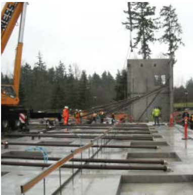
TILT-UP PANEL ERECTION
