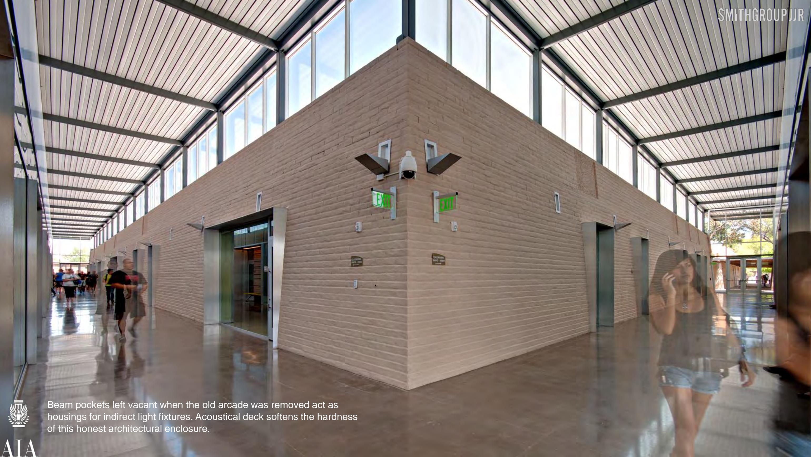
Beam pockets left vacant when the old arcade was removed act as housings for indirect light fixtures. Acoustical deck softens the hardness of this honest architectural enclosure.
